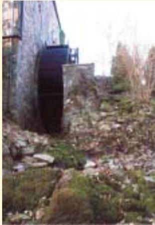
The first plan was to drive a generator with the 14ft waterwheel. However the wheel required new modern bearings and was far too noisy for 24 hour a day use. It was therefore decided to take water from the mill lade in a pipe past the wheel and down to a turbine at the side of the Shirmers Burn. The turbine would drive a small generator and with a fall of 7 meters and a flow of 100 litres per second, should produce 3kWs 24 hours a day. Hopefully
